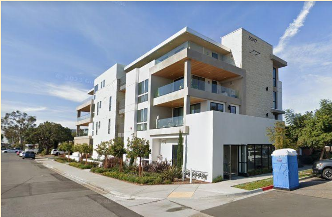
Multipurpose building on Madison and Oak Avenues
