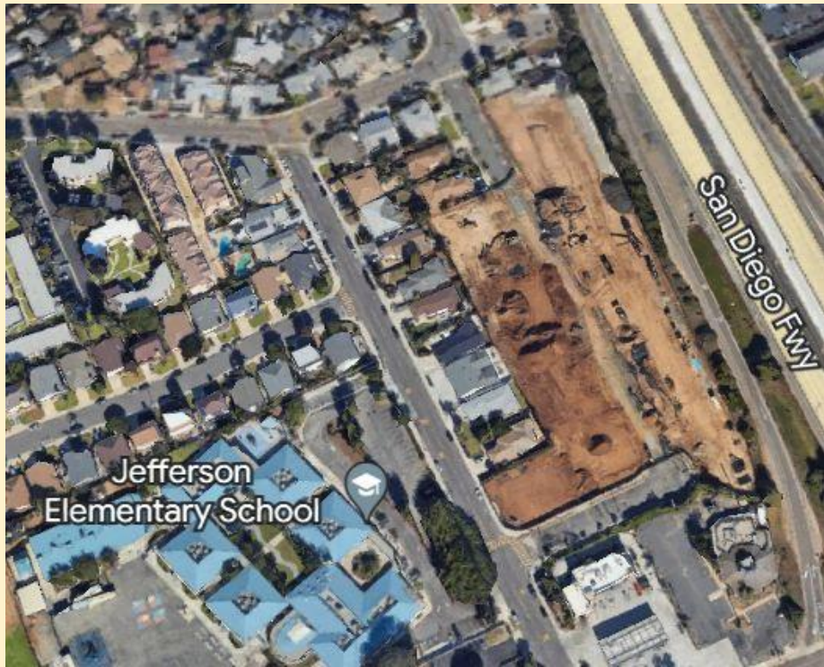
Construction along former Carol Place Street
