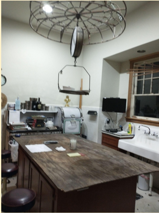
Kitchen under renovation
